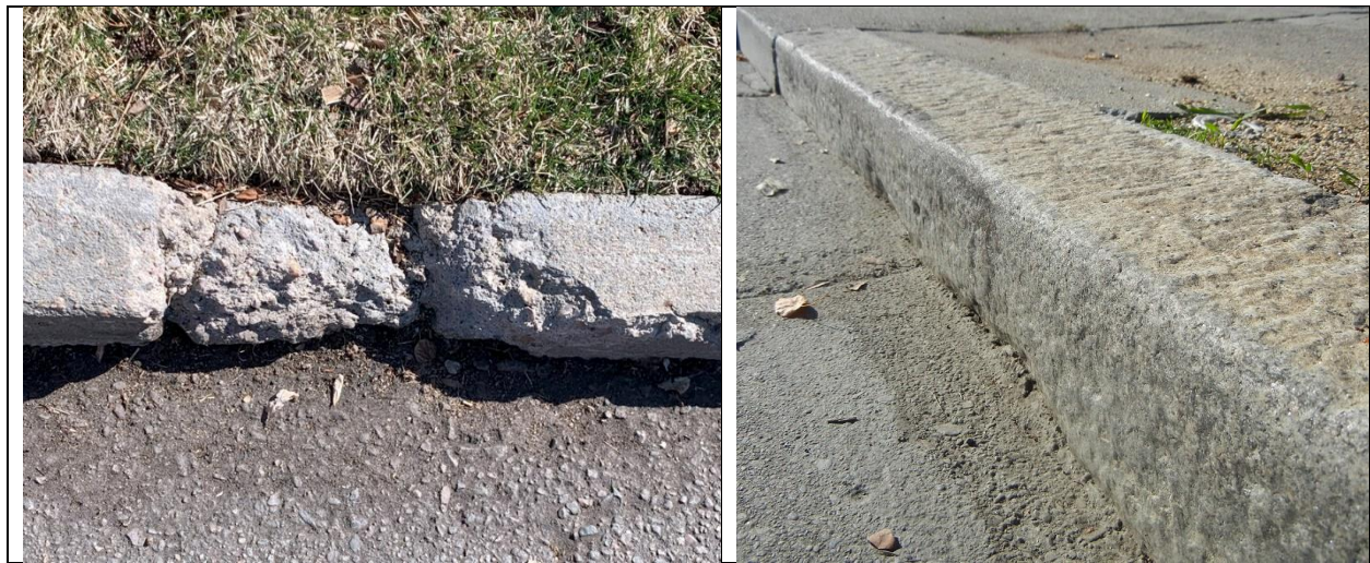
Figure 2 Prematurely Deteriorated PCC Curb vs a Century-Old yet Visibly Intact Granite Curb (Source: Denver Blog at Reddit.com and Oaklandunderfoot.com )
