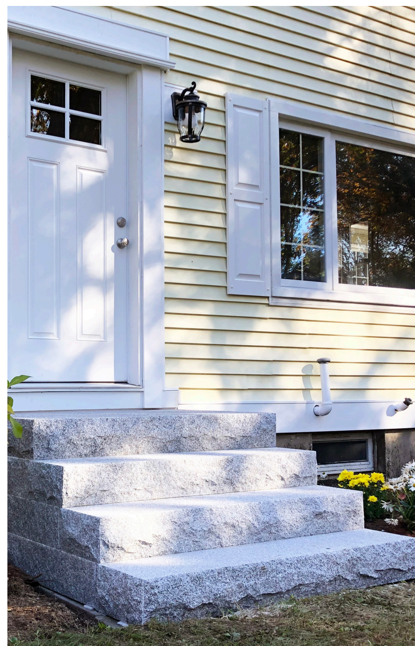
WOODBURY GRAY™ granite thermal top, rock face steps
